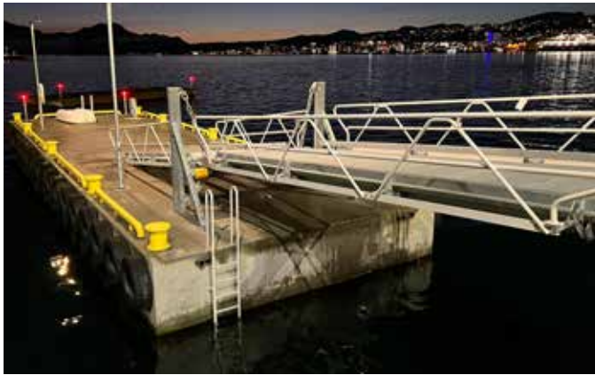
Imes Eiendom AS, Tromsø: A robust quay measuring 6 x 22 m, with a 1,2 m freeboard, and a drivable gangway measuring 3 x 13,5 m rated for a 4-tonne axle load.
