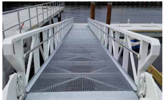
Skanska Norge AS - Nyhavna Fire Station: Gangway 20 m long, 2 m wide and supplied with steelgrating. Painted finish with CombiCoat® protection.
