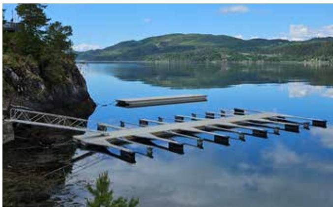
Høya Hytteforening, Levanger Municipality. Classic breakwater, concrete pontoons, walkable fingers and booms.
