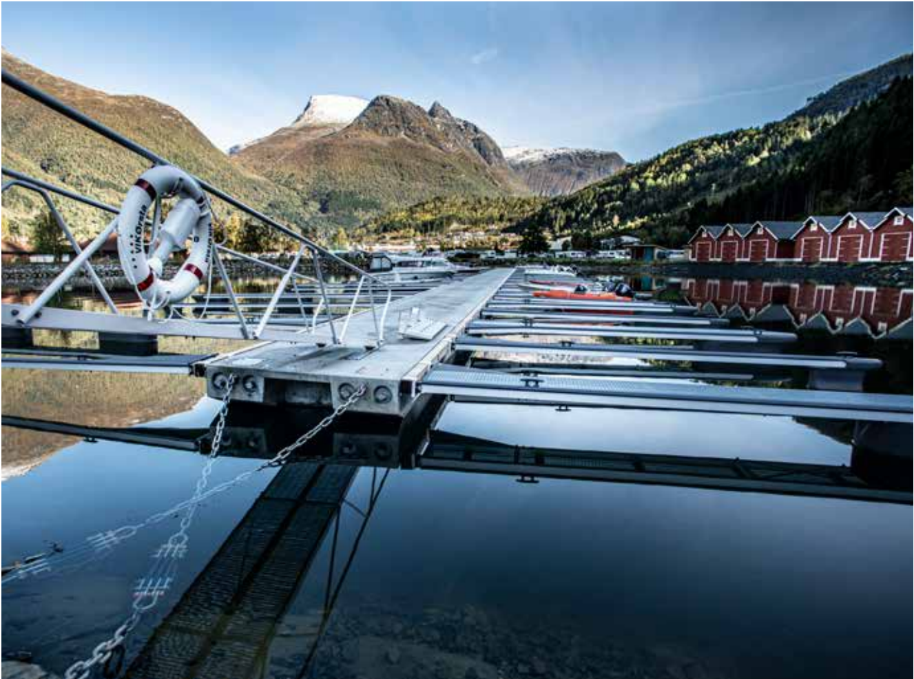
The marina at Loen Båtlag in Nordfjord features an 82-meter Ørsta Futura floating concrete pier, Ørsta Futura walkable fingers, booms and an 8 meter gangway with non-slip grating deck.
