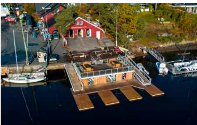
Strand Kajakk-klubb, Høvik, Bærum Municipality. Floating kayak house composed of concrete pontoons equipped with a house for storing 60 kayaks with terrace on the roof.
