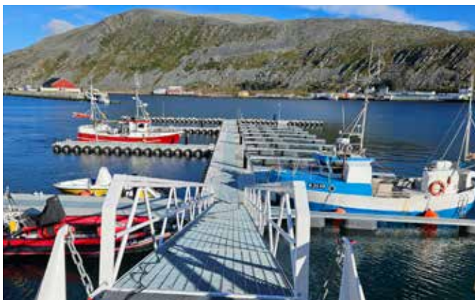
Kjøllefjord, Lebesby Municipality. Concrete pontoons with snow-free walkway and tire fendering. Gangway 14 m with snow-free grating, dimensioned for driving with ATV.
