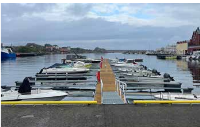
Sirevåg Havn in Hå, Rogaland County. Marina with Classic concrete pontoons, Classic steel pontoons, walkable fingers and booms.
