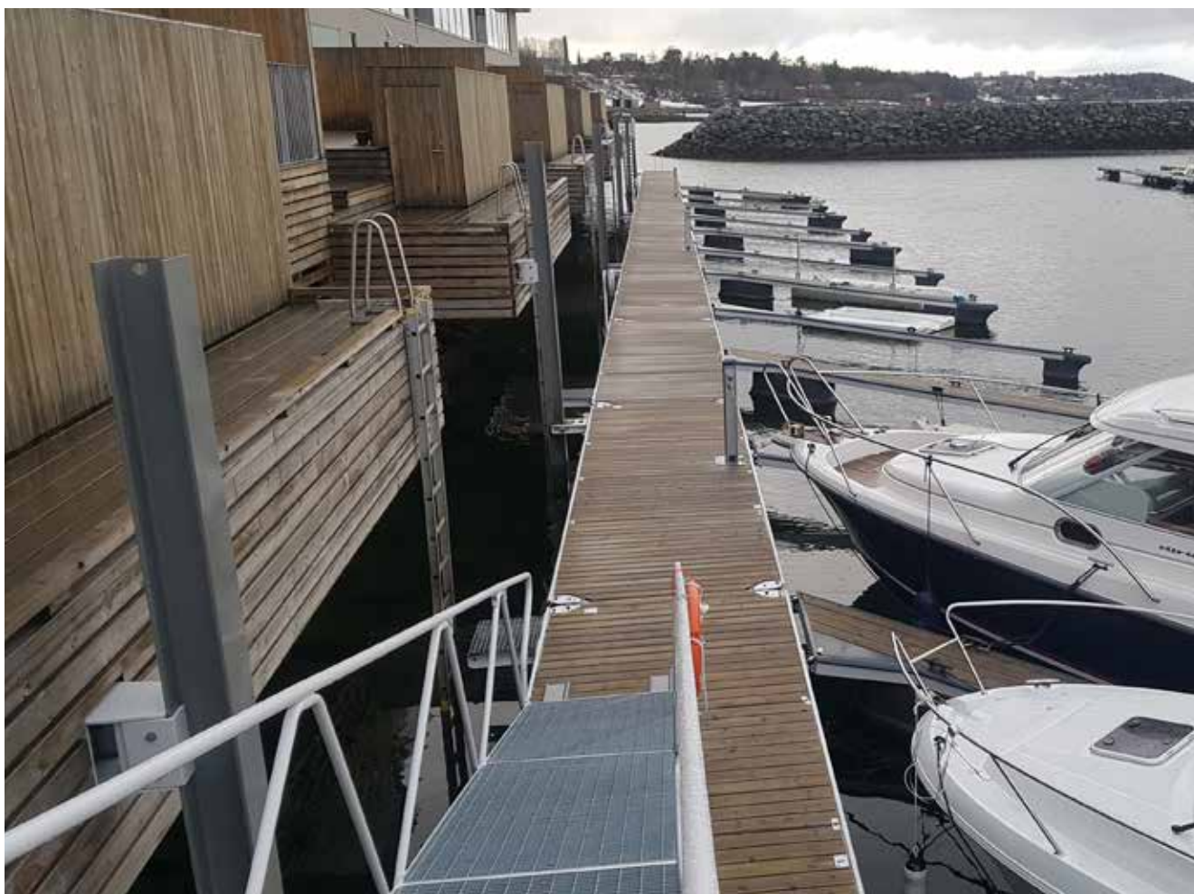
Grillstad Marina AS, Trondheim Municipality, Trøndelag county. Walkable fingers and mooring booms with an angle that ensures efficient use of space in the marina.
