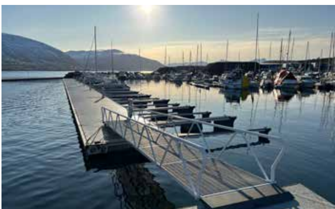
Skattøra Marina, Tromsø Municipality. 100 m breakwater with mounted pier profile that provides full flexibility in the installation of walkable fingers and booms. Gangway with grating.
